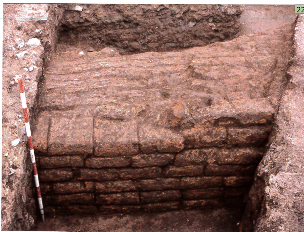
Fig. 19 Lower sewer in the interior of the amphitheatre. Brick arch.
